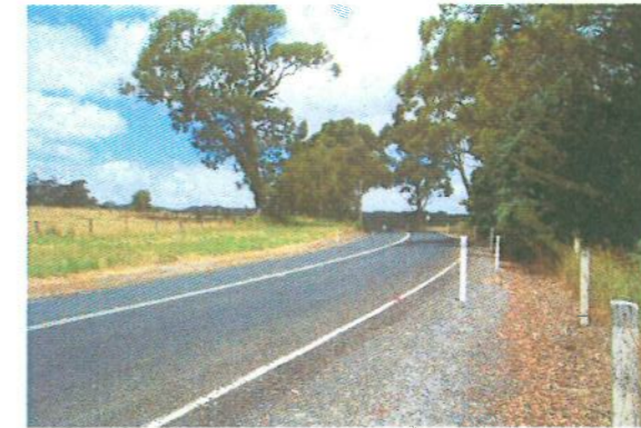
Nairne Road at Hutchens Road extension
