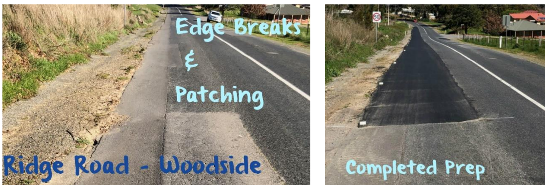
Woodside – Targeted Pavement Works – Before and After
