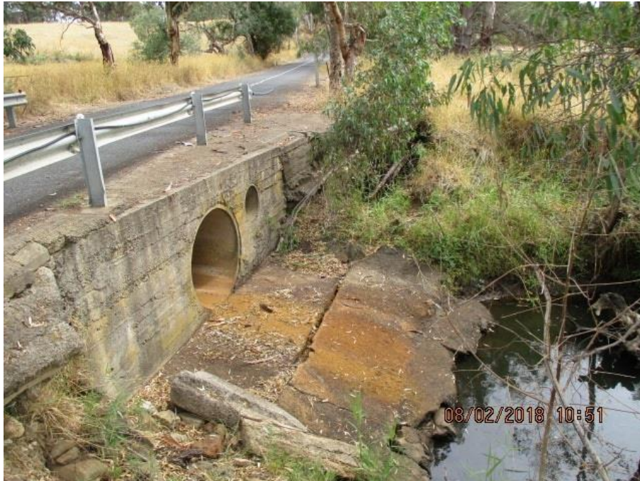
Martin Road Pipe Bridge - Oakbank
