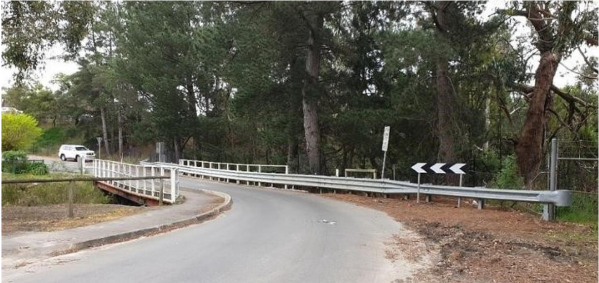
Onkaparinga Road – Bridgewater Span Bridge
