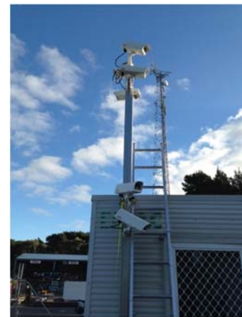
Windmill Hill Transfer Station System Upgrade
