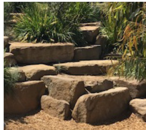
Boulder edging and steps to reservoir softfall
