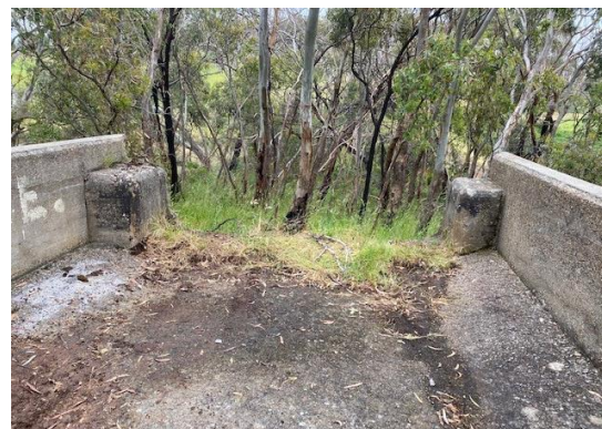
(b) Northern approach (view from deck slab)
