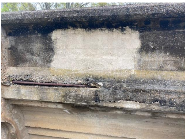
(a) Eastern Parapet Wall
