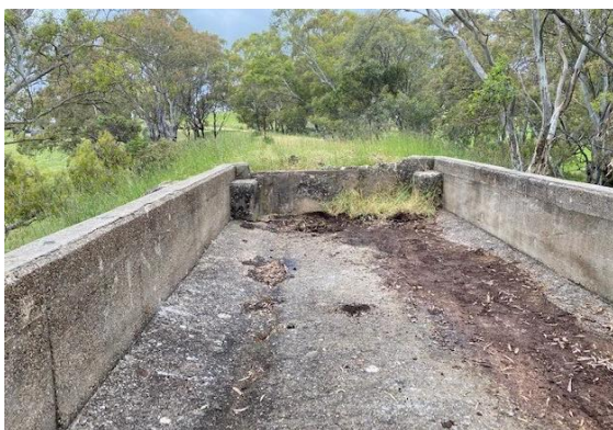
(a) Southern approach (view from deck slab)
