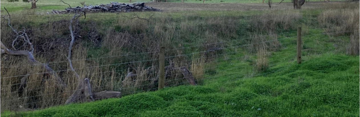
Figure 2-2. Electrified fence encountered during site walk-over
