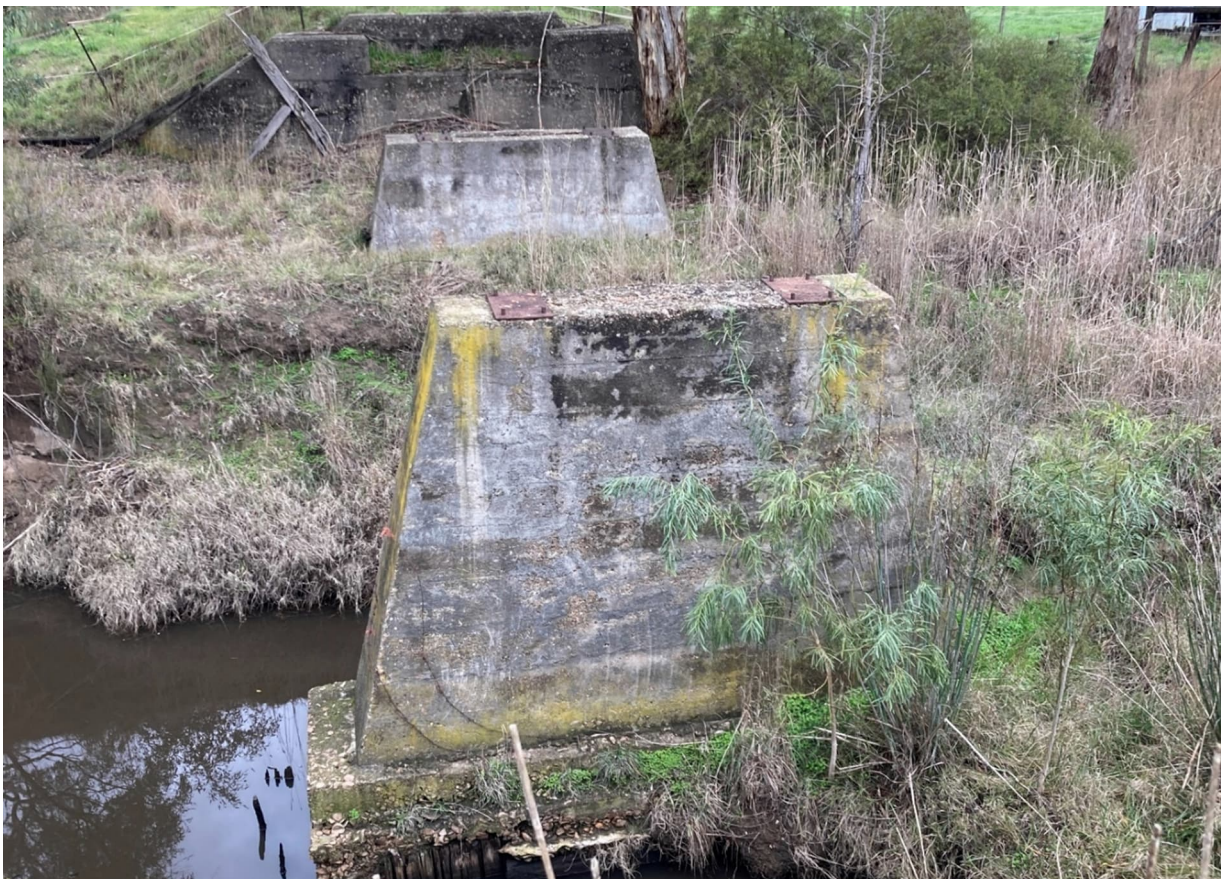
Figure 2-5. Angas Creek railway bridge piers and northern abutment (looking south)
