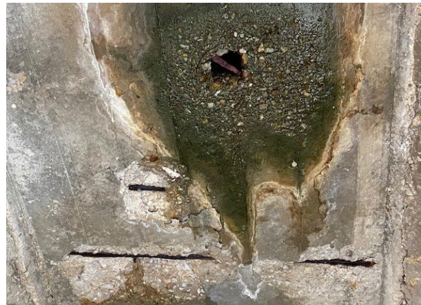
(b) Deck soffit near northern scupper
