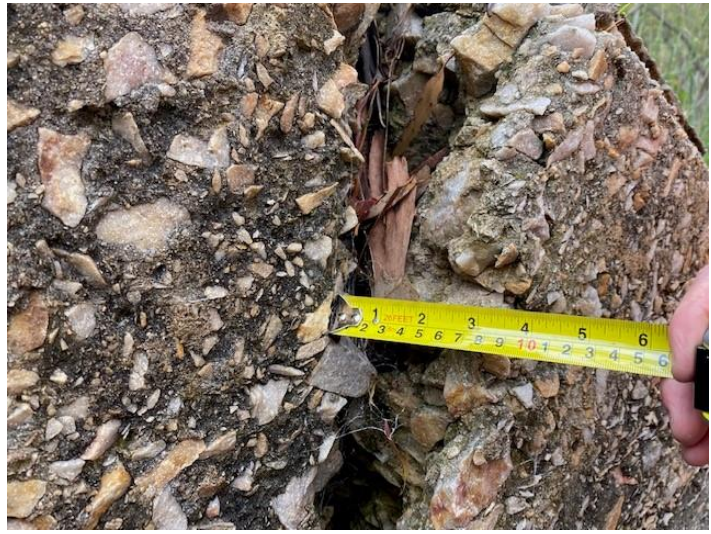
(b) 70mm crack width
