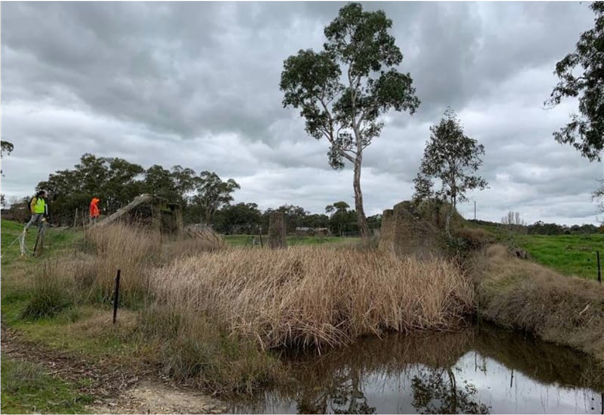
Figure 2-4. Williams Creek railway bridge abutment, wingwalls and pier (looking east)
