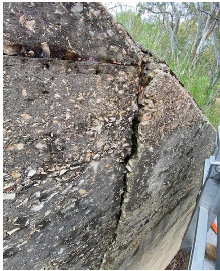
(a) Rotation of Southeastern Wingwall
