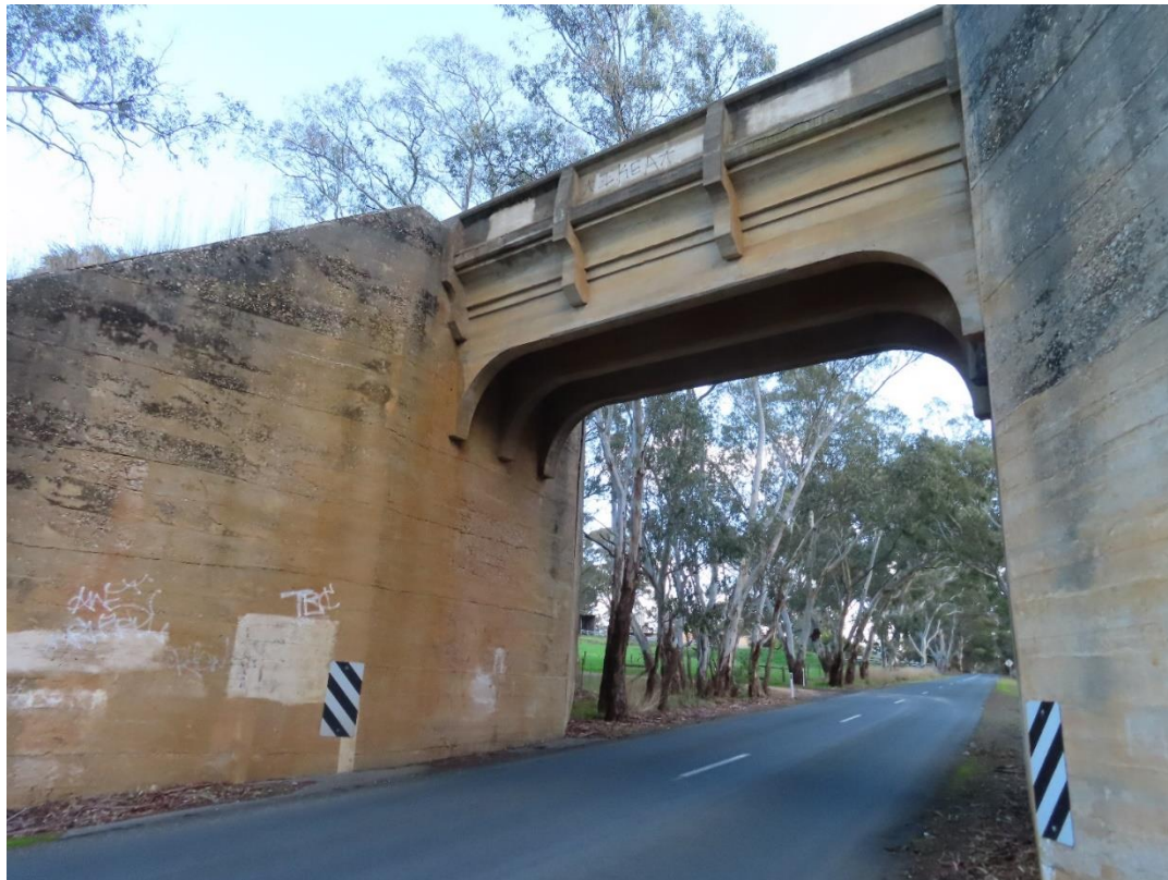
Figure 1 The Existing Burfords Hill Road Bridge
