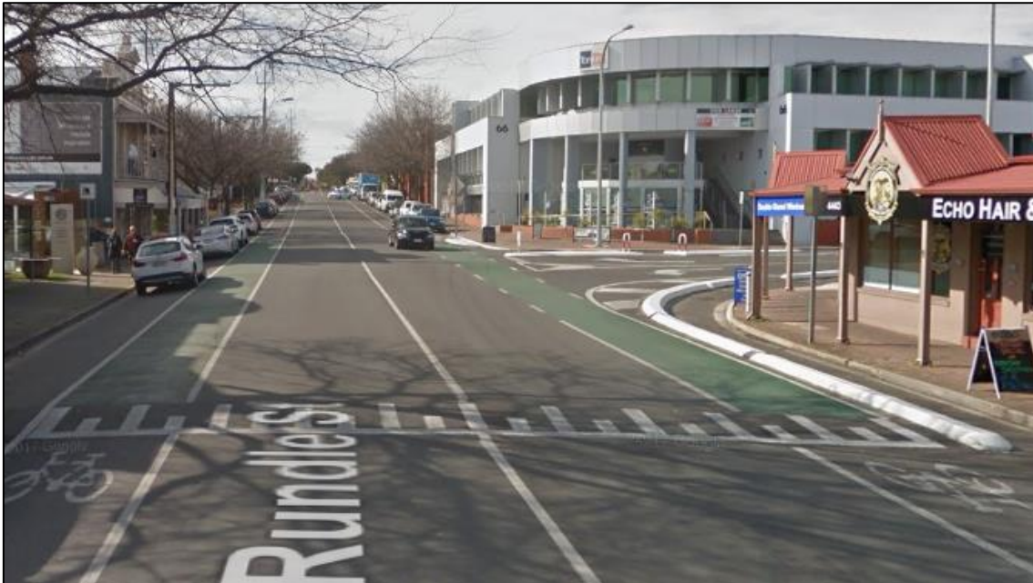
Figure 7: Raised Intersection Pavement
