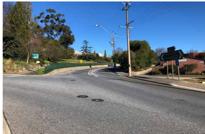
The western entries to Albert Street are wide and promote high vehicle speeds.
