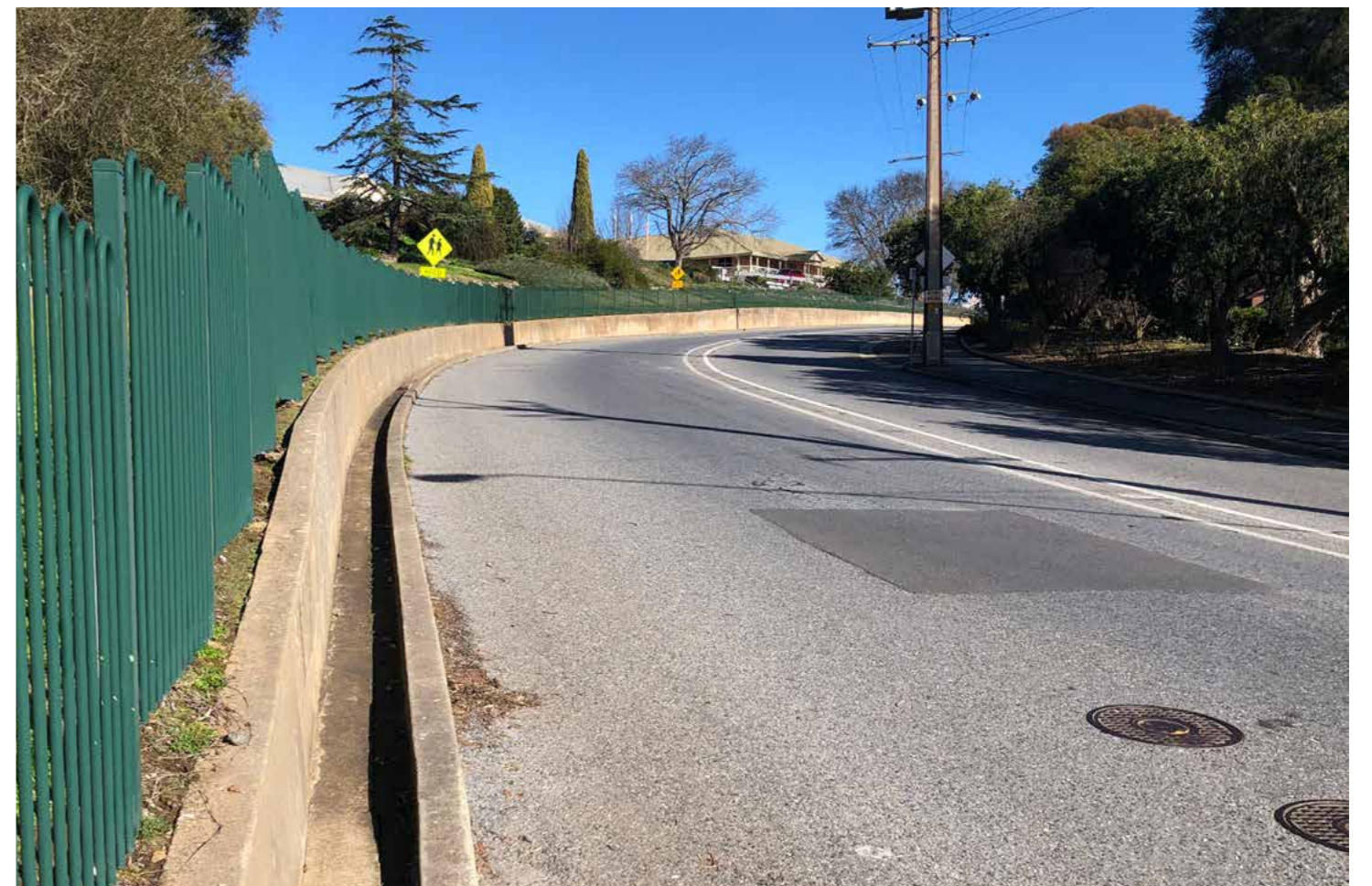
Length of concrete retaining wall to Memorial Hospital is an opportunity for public art and an entry statement to Albert Street.
