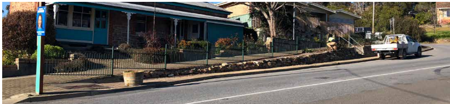
Gumeracha Main Street is on a steep slope with minimal stormwater infrastructure.
