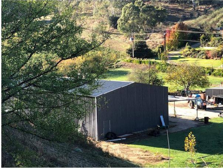
Photo 4: Existing farm shed at the front of the site
