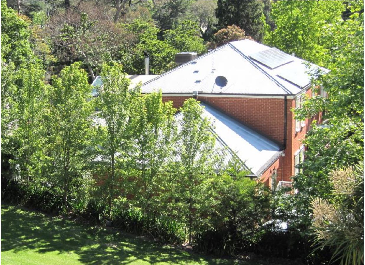
Image 1: Dwelling at 18 Pomona Road as viewed from the subject land.
