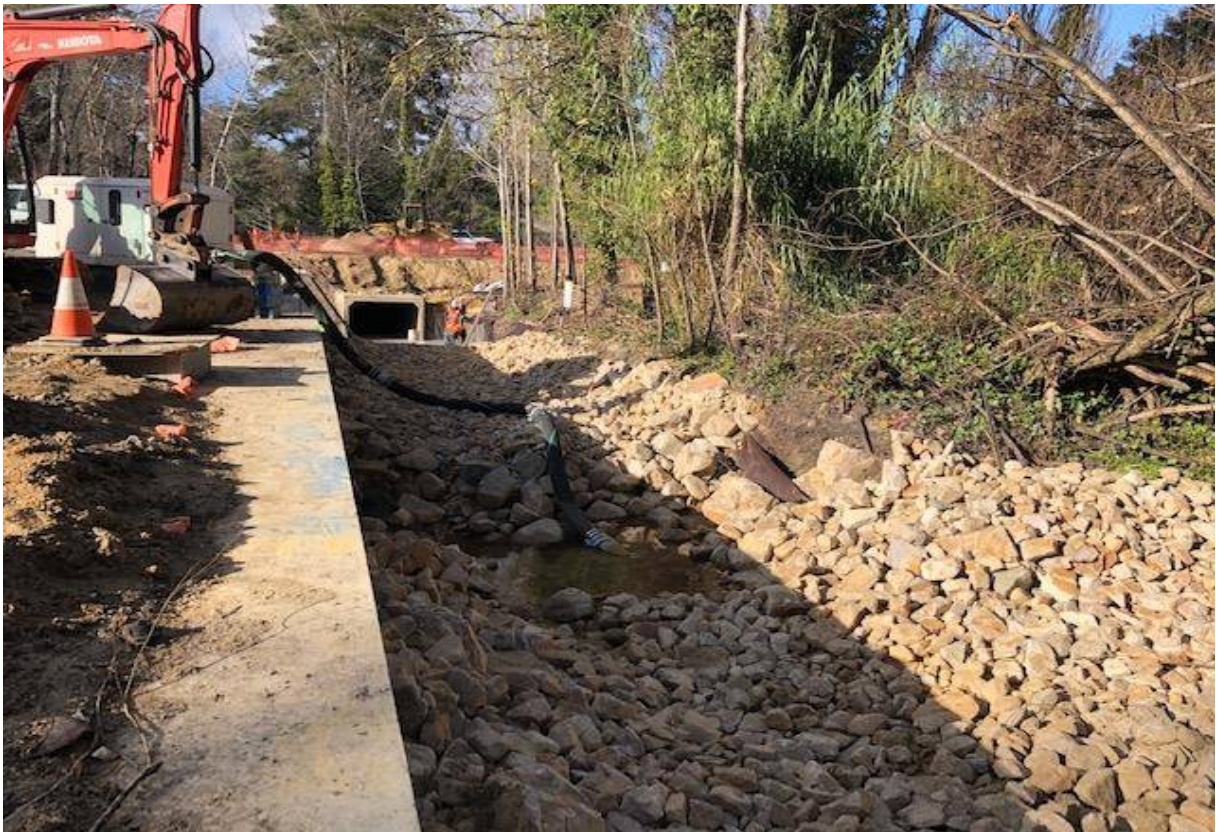
Photo 4: Rock lined creek channel and building foundation– Aldi site
