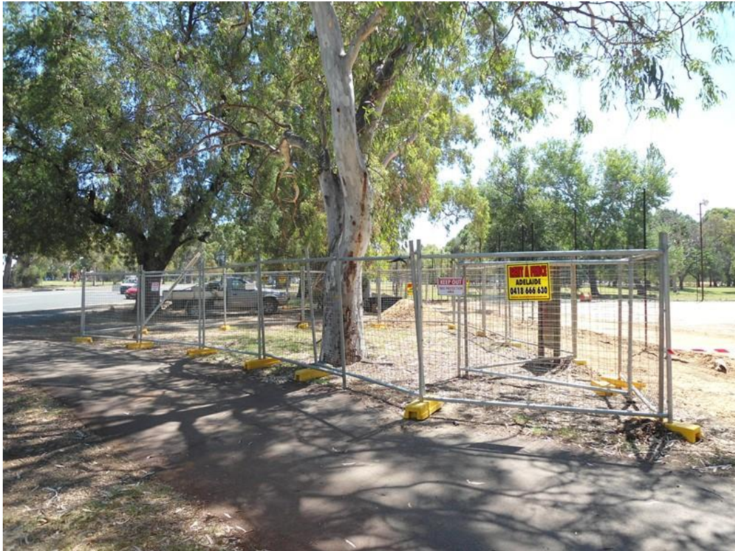
Figure 2: Typical TPZ fencing
