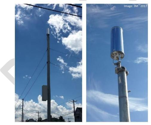
Figure 6: Reflective wrap installed on antennae to reflect background and respond to changing light conditions
