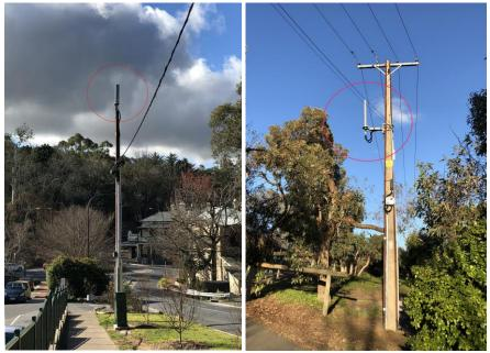
Figure 1 & 2: Current 4G installations with omni antenna on utility pole and ground based enclosure (Aldgate and Bridgewater installation)
