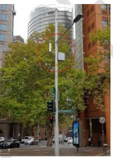
Figure 3: Current 4G installations using a "Koala" equipment enclosure on the pole (no ground based cabinet)
