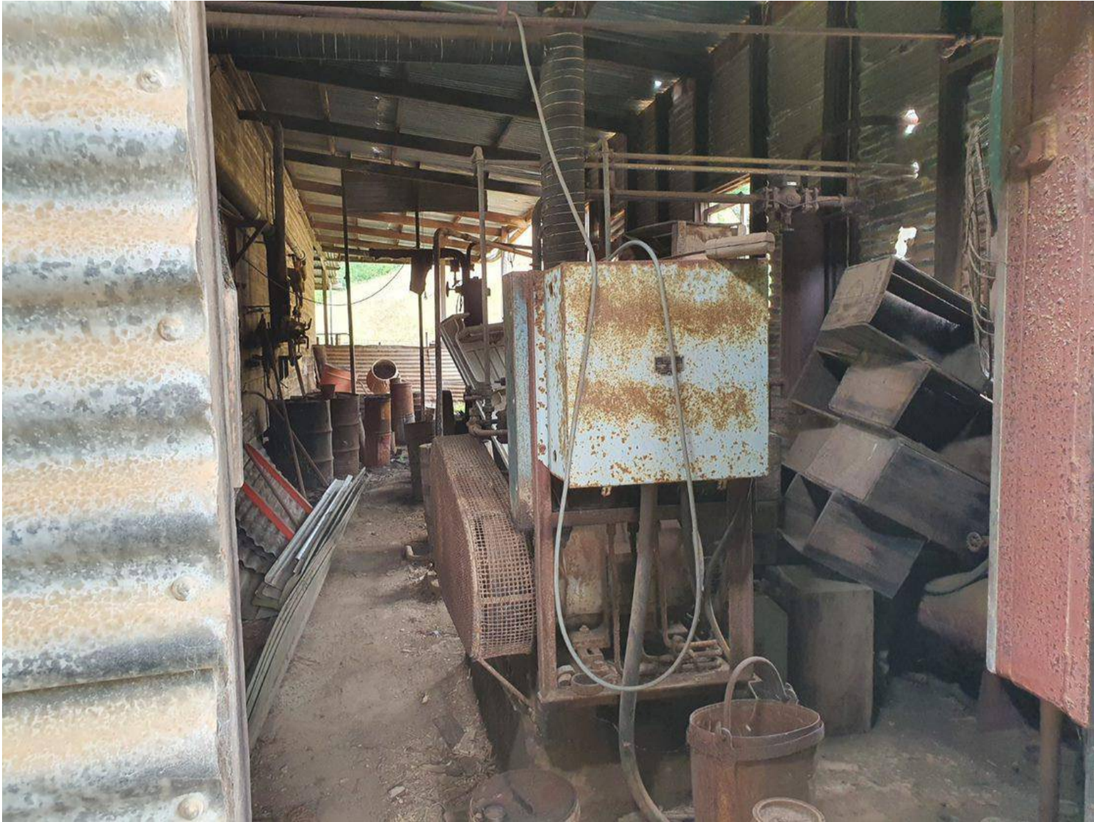
Description: View of old generator next to wooden storage shed
