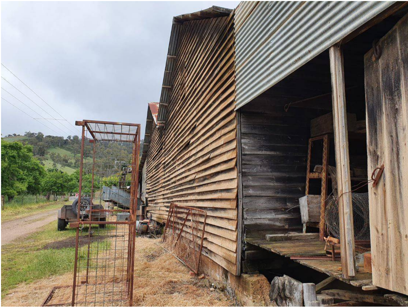
Description: View of outside of wooden storage shed
