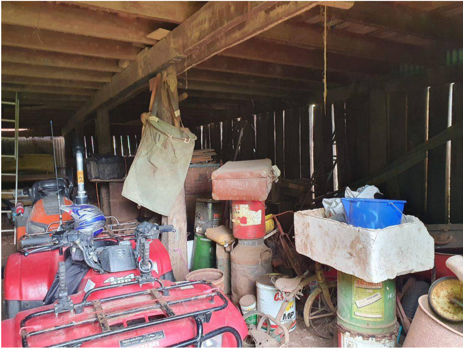
Description: View inside first wooden storage shed
