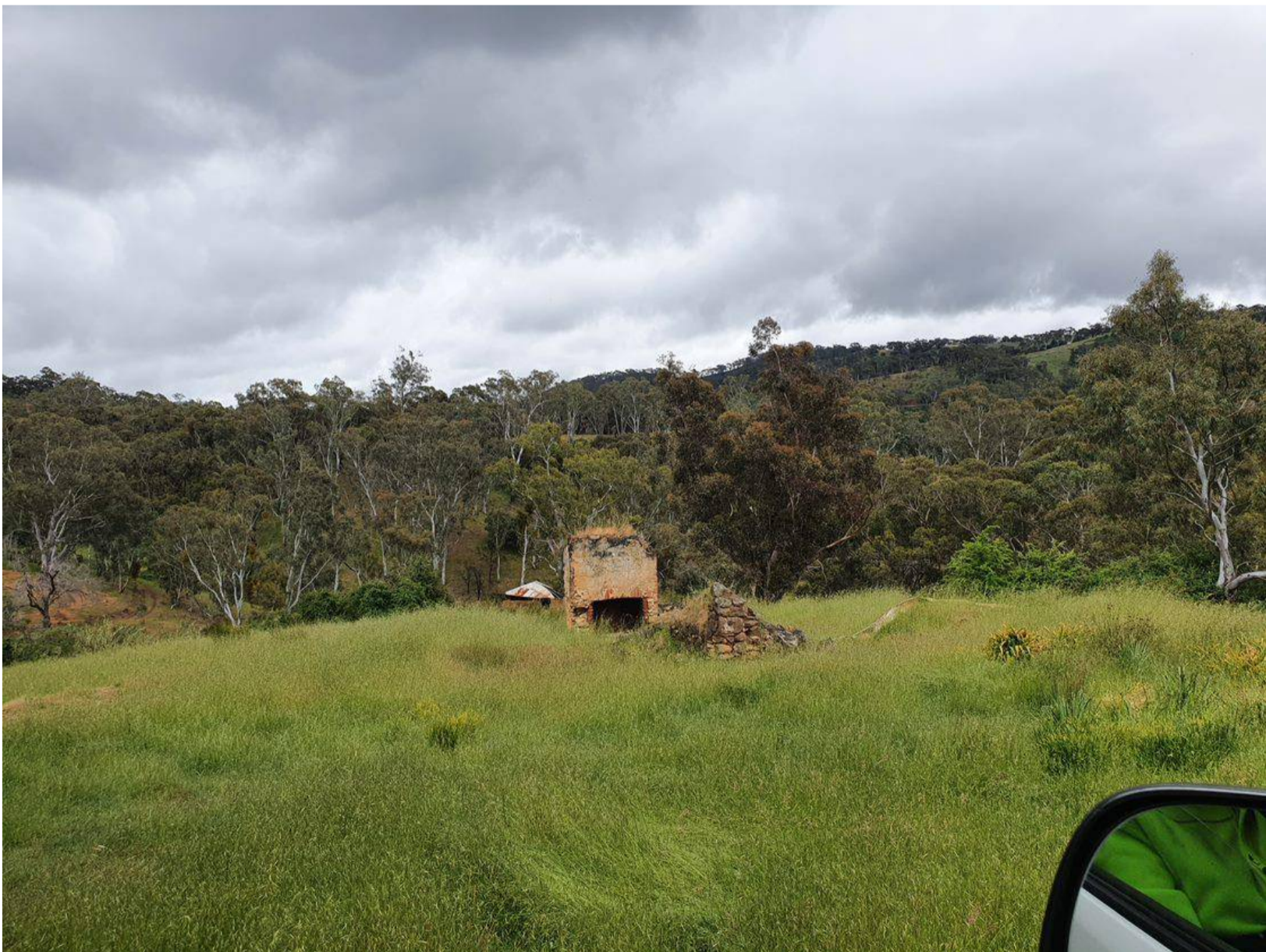
Description: View of former house (ruins) in western portion of site
