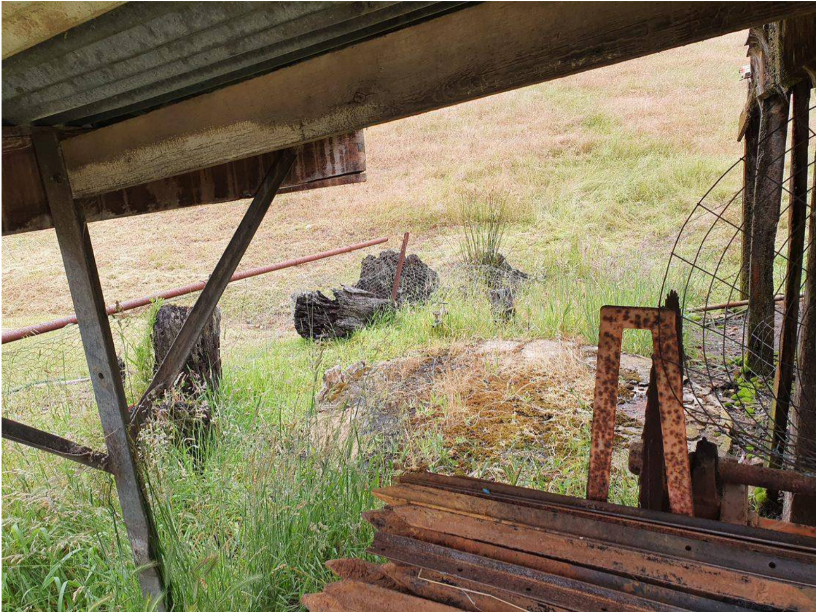
Description: View of concrete pad for former tank at the spray shed
