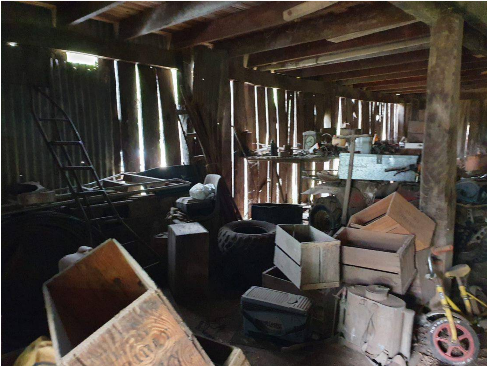
Description: View inside first wooden storage shed
