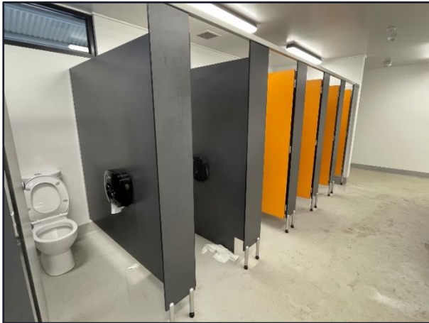
Wet area, Home change room
