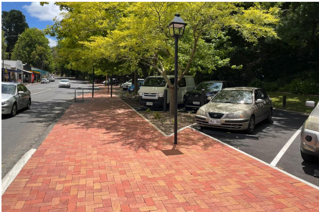
Recently Completed Aldgate Main Street Amenity Upgrade – Stage 1
