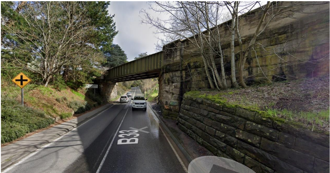
Aldgate Railway Bridge [currently] – Aldgate to Stirling
