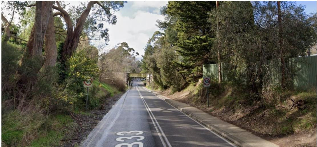
Aldgate Railway Bridge [currently] – Stirling to Aldgate
