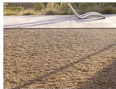
Compacted Sand / Gravel Paving
