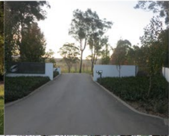
SIGNAGE AND ACCESS GATE
