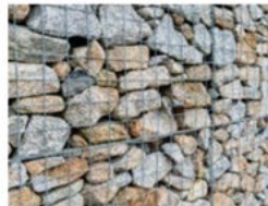
W1 - Gabion Wall - Local Stone
