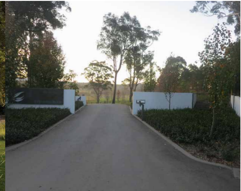
SIGNAGE AND ACCESS GATE
