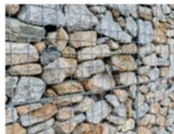
W1 - Gabion Wall - Local Stone
