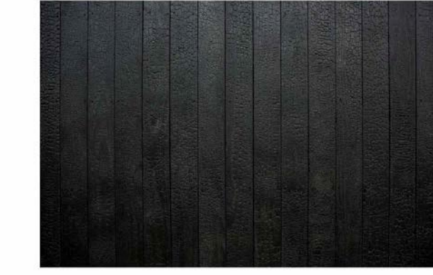
CLD-1A_ CHARED TIMBER SHIPLAP CLADDING
