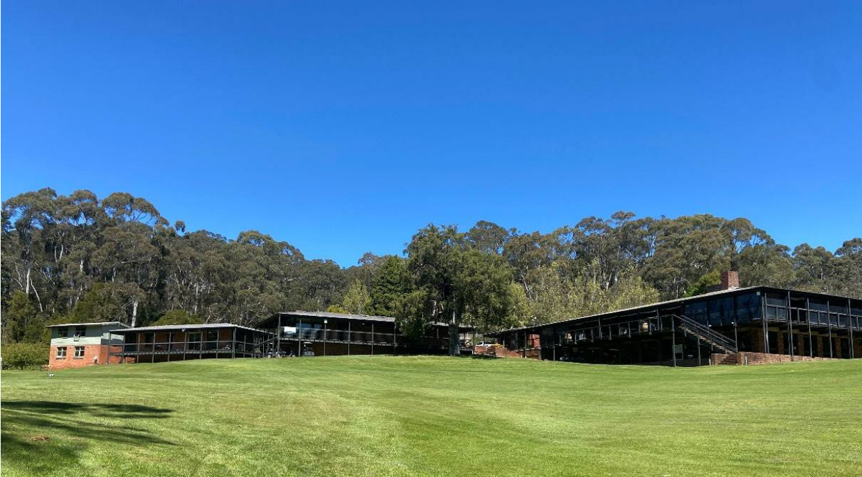
Image 2 – Existing Clubhouse Buildings
