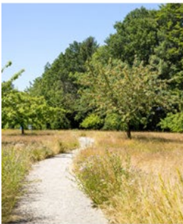
P1 - COMPACTED GRANULITIC PAVING
