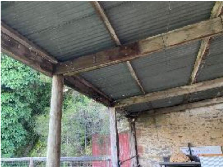
Replace timber purlins throughout spaced at 900 centres and capable of spanning 3000mm to support roof.
