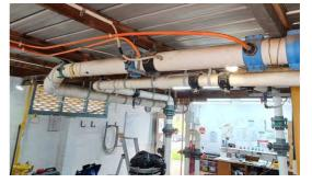
Figure 30: Dosing Points into Filtered Water Line
