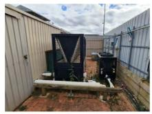
Figure 34: Electric Heat Pumps
