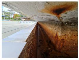
Figure 11: 25m Pool North Scum Gutter
