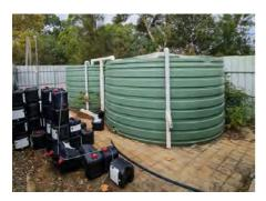
Figure 19: Backwash Holding Tanks
