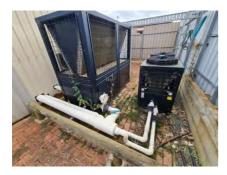
Figure 33: Electric Heat Pumps
