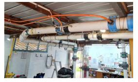
Figure 30: Dosing Points into Filtered Water Line
