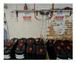
Figure 27: Sulfuric Acid Dosing Pumps & Carboys
