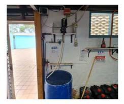
Figure 28: Sodium Bicarb Dilution Tank & Dosing Pump
