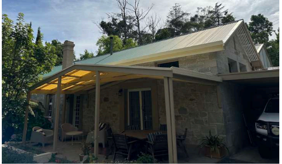
Figure 8 – Former Coach House, West Elevation
