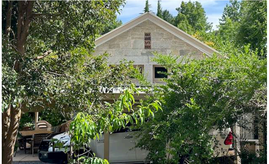
Figure 19 – Former Coach House, gable end of South Elevation should remain visible
