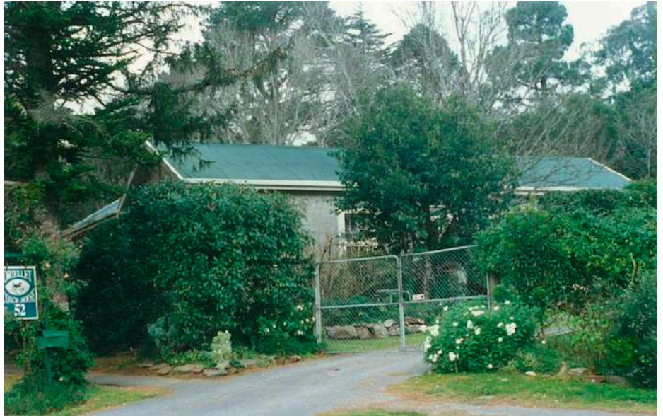
Figure 7 – Coach house, 1996 [Source: Weidenhofer 1997:STI52]
