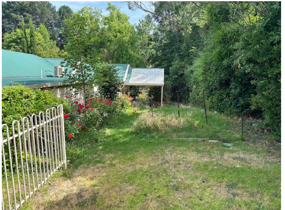
Figure 13 – Former Coach House, East Elevation
