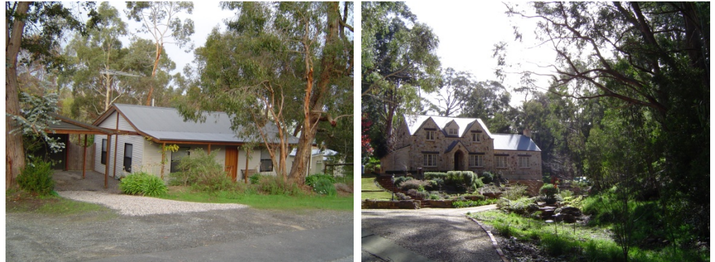
The use of iron, timber and stone should be encouraged.
