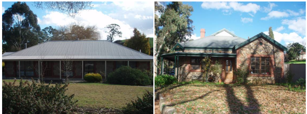
Photos 9 & 10: The majority of more recent dwellings feature hipped rooves, verandas, are of stone or brick construction and are set well back behind substantial front gardens.
