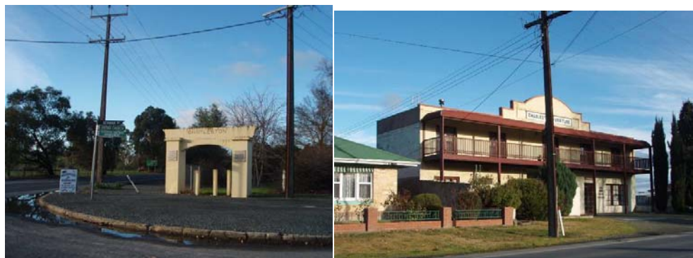
Photos 7 & 8: Landmark buildings are limited within Charleston.
