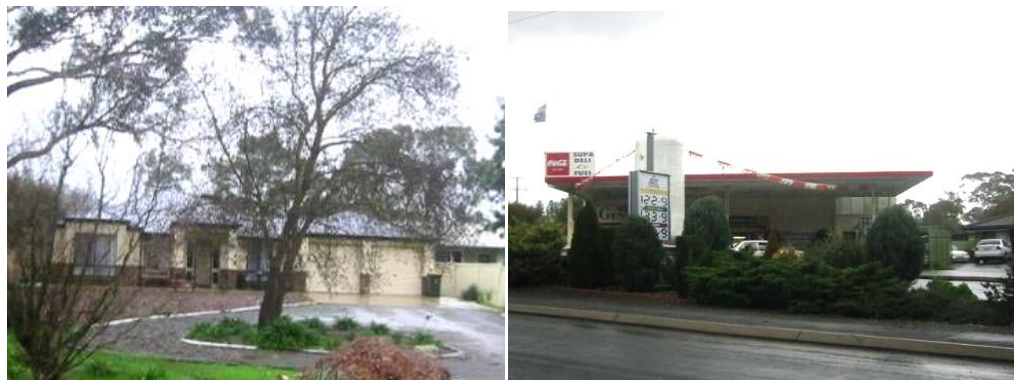
Photos 1 & 2: Kersbrook is predominantly a very low-density residential township with a local centre service function.
