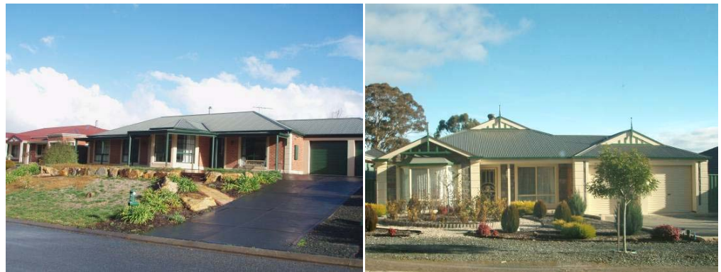
Photos 9 & 10: More recent residential development features hipped rooves with modest verandas and brick construction
