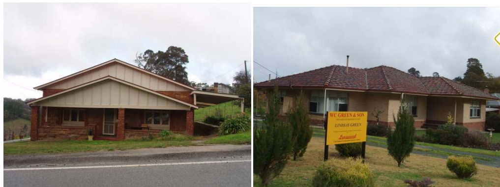
Photos 5 & 6: Building styles feature pitched rooves with brick walls and either tiled or colourbond rooves.
