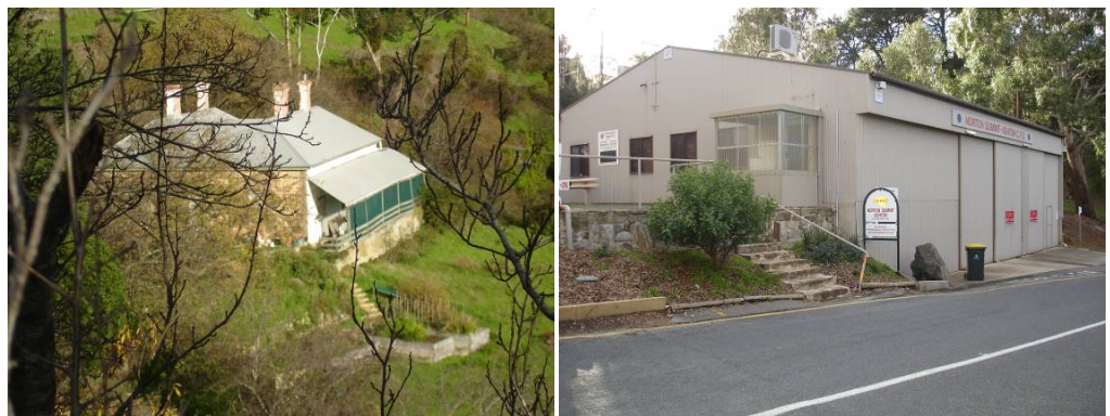
Photos 7 & 8: Building design varies from historic dwellings to more recent structures.
