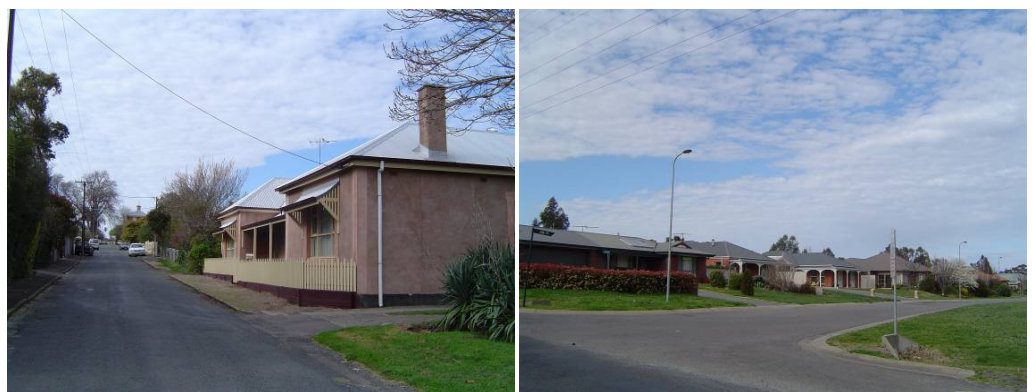
Photos 3 & 4: The older portions of Oakbank feature narrow north-south orientated streets, upright kerbs and gutters, footpaths, overhead wires and minimal setbacks to buildings. The newer portions feature wider roads, roll-over gutters, no footpaths, underground wires and large setbacks to buildings.
