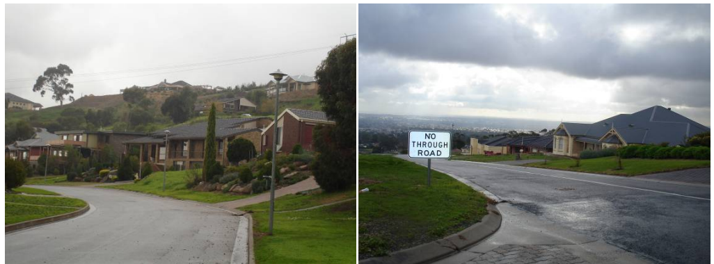
Photos 3 & 4: The road layout is based on a single collector road with smaller cul-de-sacs feeding off it.
