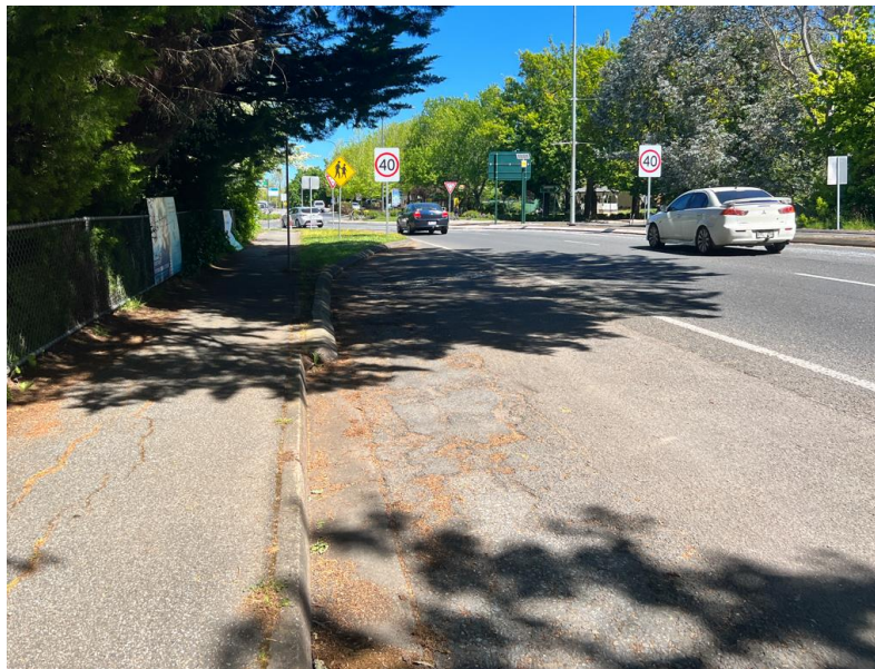
Figure 16 - Looking south at the proposed space
