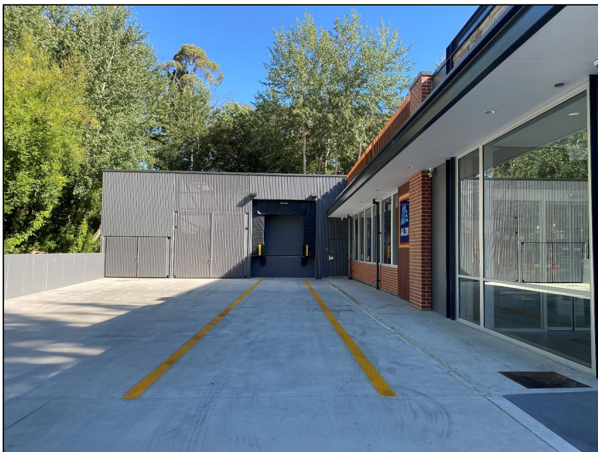
Figure 4: Existing loading bay within the ALDI car park
