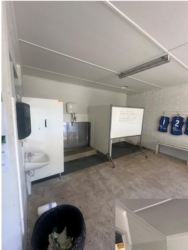
Image 3- AWAY Changeroom Area (open shower behind whiteboard)
