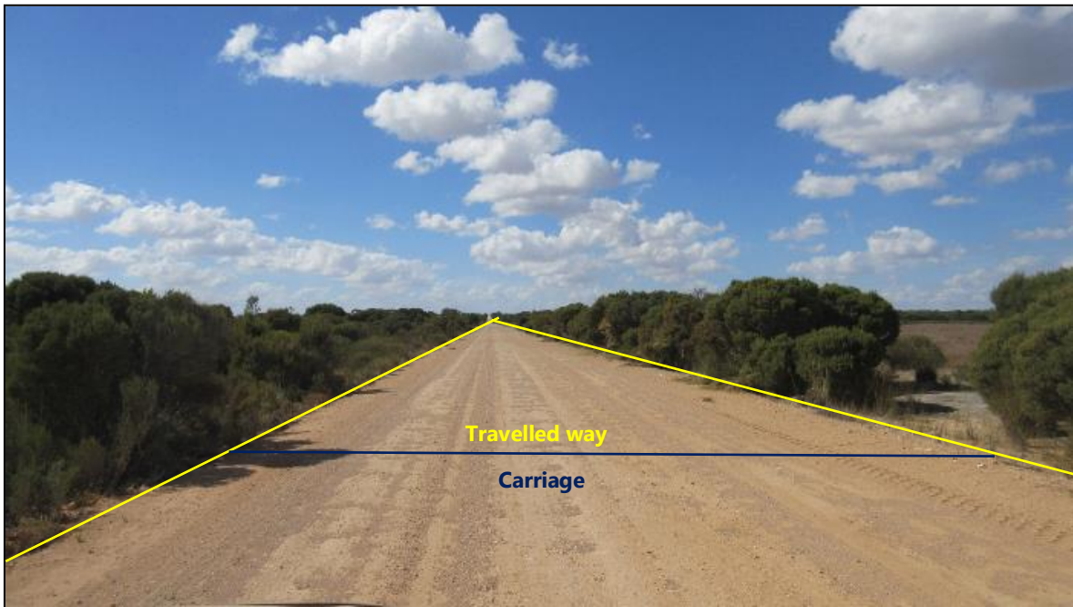
Figure 8: In this instance the carriageway has been created at a width where there is only remnant vegetation remaining on either side of the road. Any clearance beyond the carriageway would require an application.
