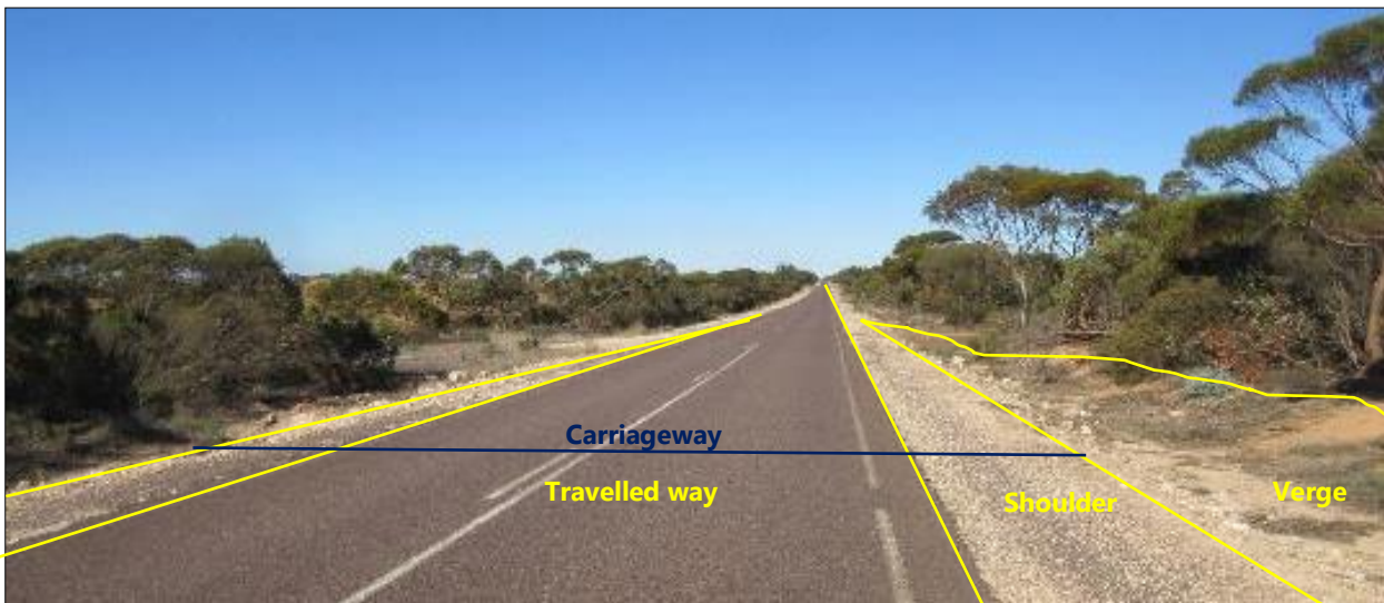
Photo 4. A rural sealed road, with an obvious shoulder and distinct verge and natural ground surface present
