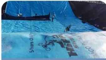
Pond liner laying
