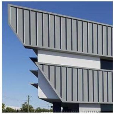
01 - STANDING SEAM CLADDING - LIGHT GREY
