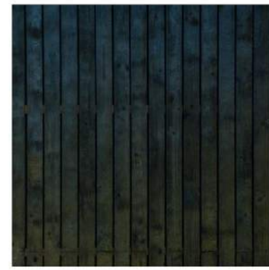
04 - CHARRED TIMBER CLADDING
