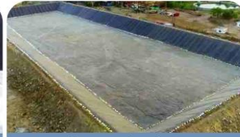
After complete laying
