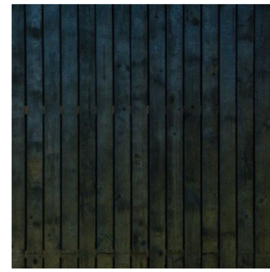
04 - CHARRED TIMBER CLADDING
