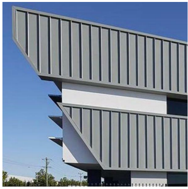
01 - STANDING SEAM CLADDING - LIGHT GREY
