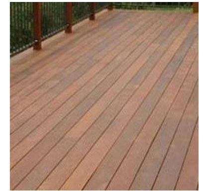
05 - TIMBER LOOK DECKING
