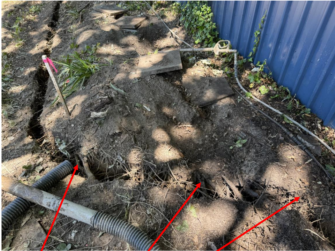
Stepping in of retaining wall
