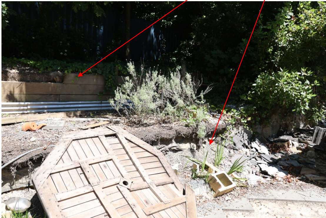
Two Levels of retaining walls, distance from boundary first level 2.8m, second level 5.3m, both are 900mm in height.
