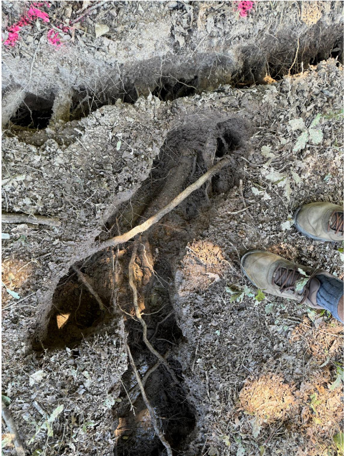
This photo was taken near the major trench to show roots extending towards the 4.1m line.
