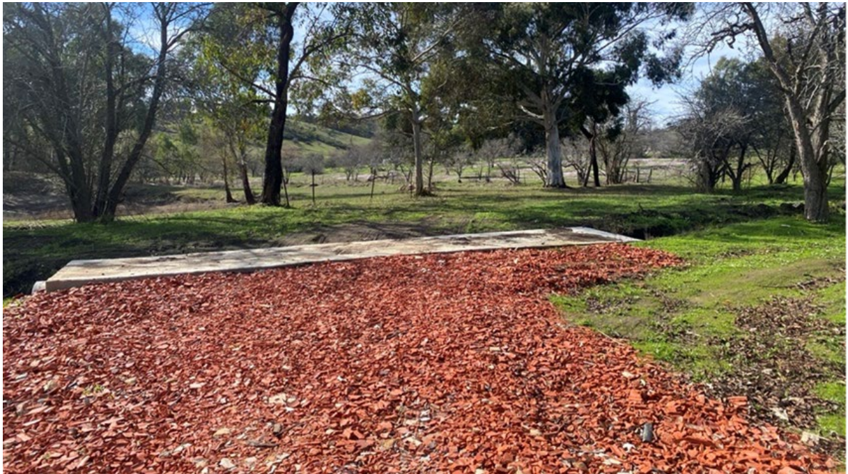
Figure 1: views to the north-west of the culvert.
